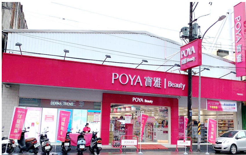
Poya Community Shop
